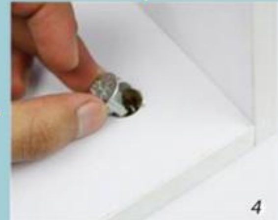
4 Insert The Eccentric Wheel Into The Round Hole
