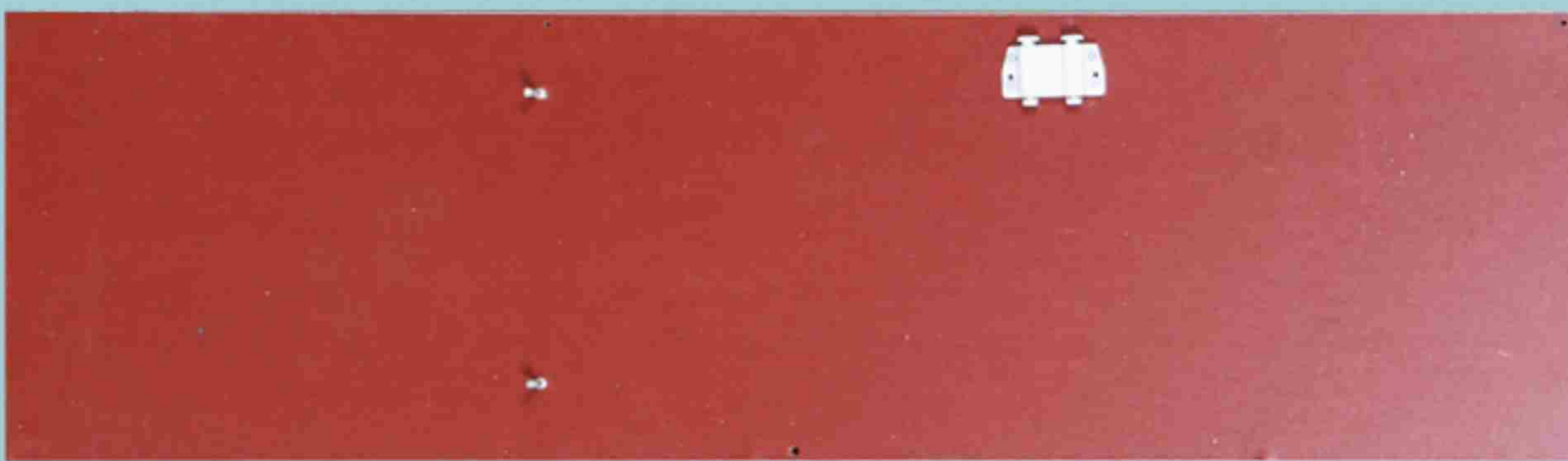
⑦ Roof plate
